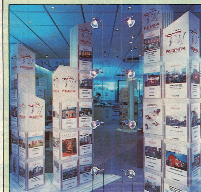
A low voltage, bare wire spotlighting system used by Prudential Property Services to light information cards in a shop window. The system allows the miniature spotlights to be positioned anywhere in the window, putting maximum light on the cards with minimum intrusion. Called Hi Wire, the system is from Hitech Lighting plc.
