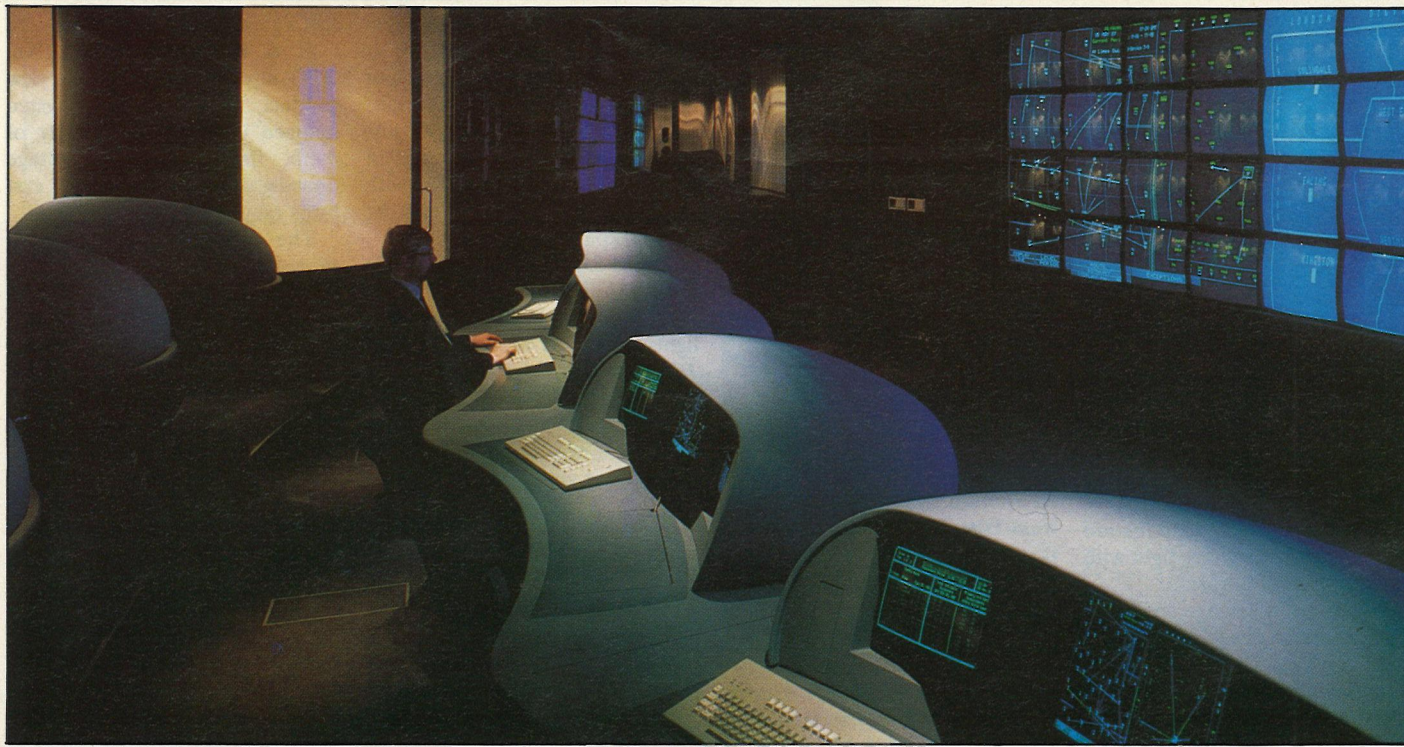
British Telecom's network management centre lit by Concord. Low voltage recessed downlights with special anti-glare baffles light VDUs.
